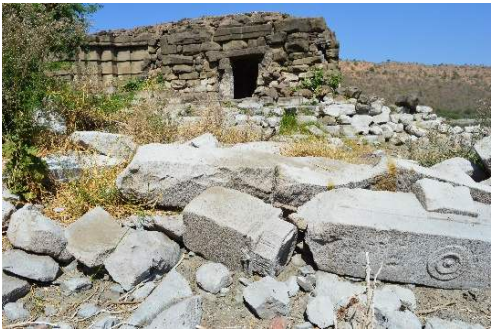
Fig. XI. The temples at the crater lake periphery are found in ruins due to the earthquake on Deccan Plateau of 1803 (Bugdane S. T. 1990).
